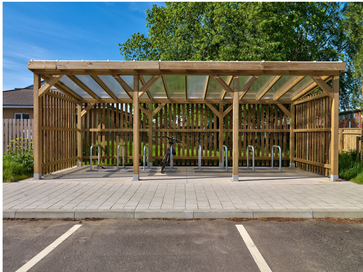
Covered Cycle Storage Area
