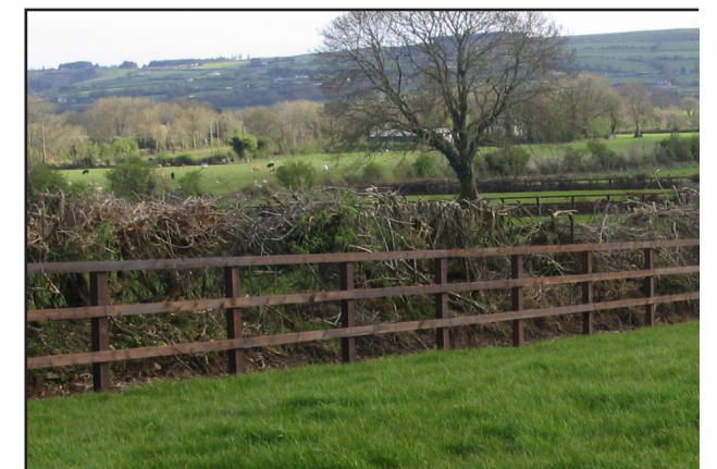
Timber Post and Rail Fence 1.4m high
