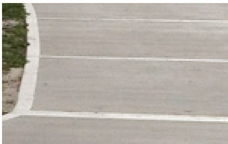
Brushed Concrete with trowel edge finish (streets)
